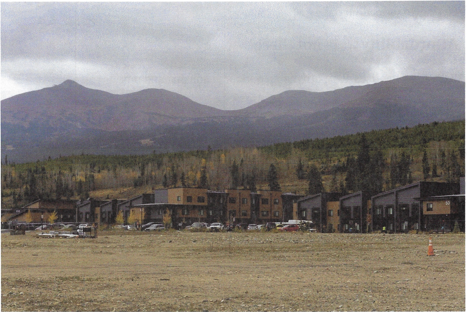
The Vista Verde workforce housing complex in Breckenridge. The complex's second phase, which opened in fall of 2024, brought 174 income-based rental units aimed at households making between 80% and 120% of the area median income.
