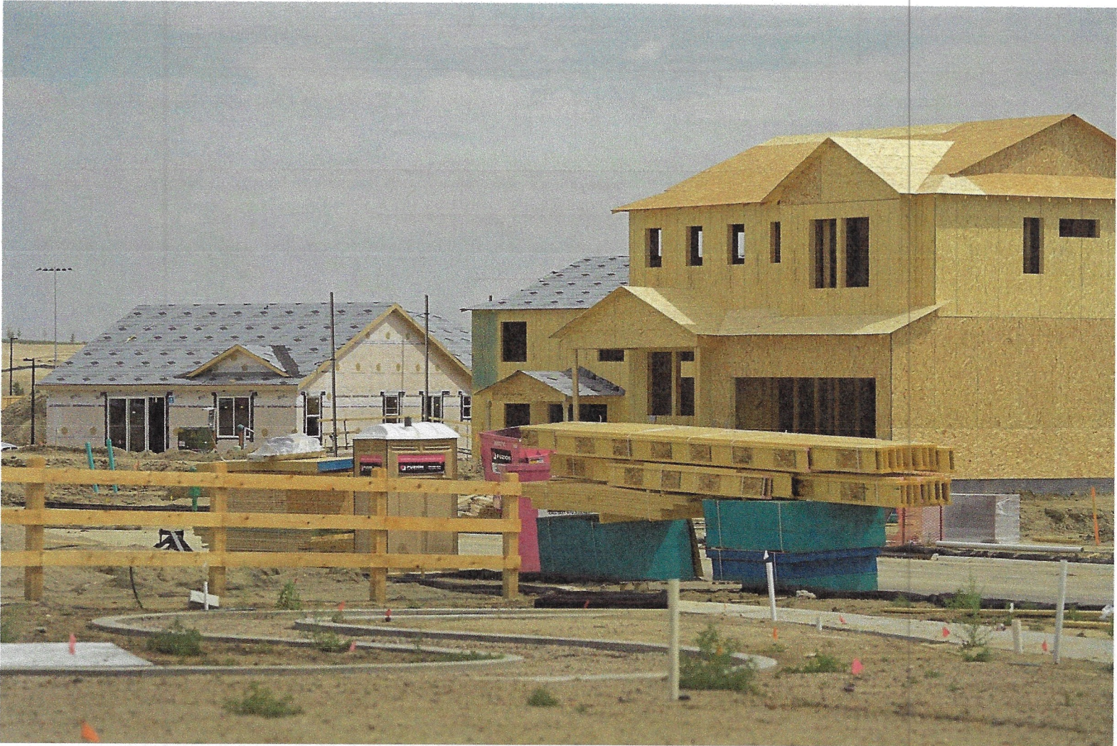
A construction site at the Looking Glass development in Parker on Wednesday. HYOUNG CHANG — THE DENVER POST
