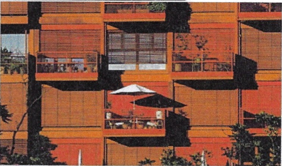
Young people seeking relief from the sweltering heat jump from a bridge into Paris's Canal Saint-Martin, above; closed blinds and empty balconies on a residential building in Berlin, below; a man on a train in London wipes away sweat, right. CLOCKWISE FROM TOP: LUDOVIC MARIN/ AFP/ GETTY IMAGES; KIN CHEUNG/ ASSOCIATED PRESS; FILIP SINGER/ EPA/ SHUTTERSTOCK
