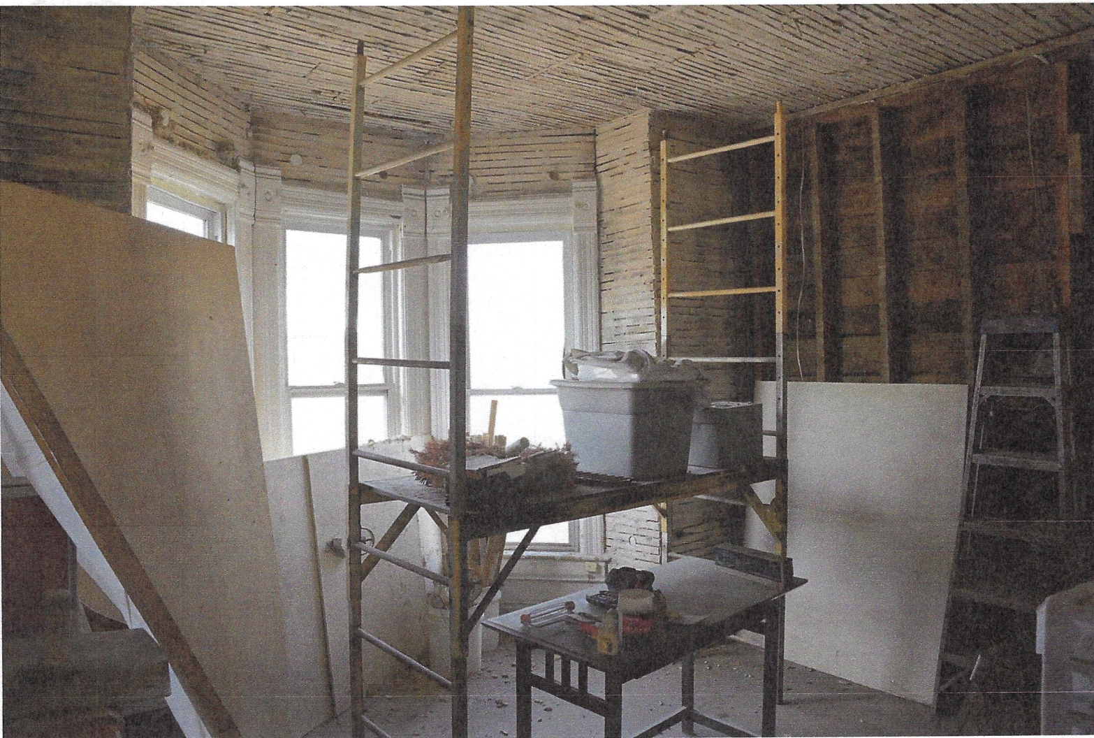
Renovations are underway Tuesday at the Sandoval family's home.
